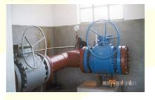
Expandable pipe connectors are set up 设有可扩展的管道接口
